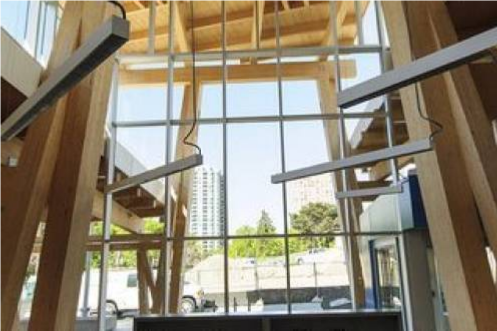
Scarborough branch interior Credit TPL
