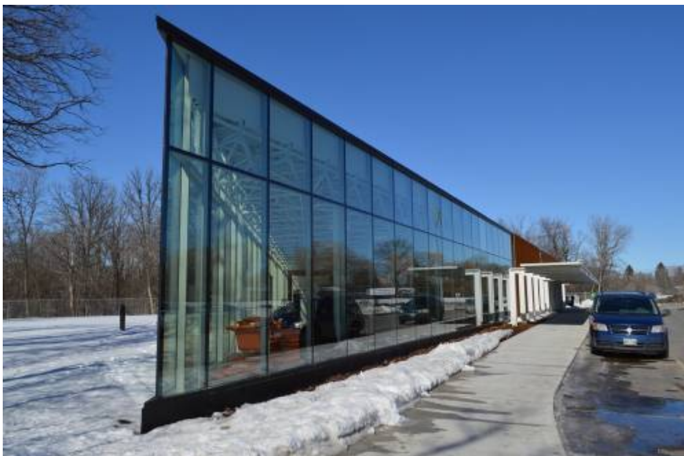
15.1 Winnipeg Public Library, Windsor Park Branch. Exterior. Credit Winnipeg...
