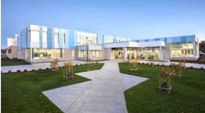
8.1 Regina Public Library, Albert Branch at mâdawêyatitân centre. Exterior...
