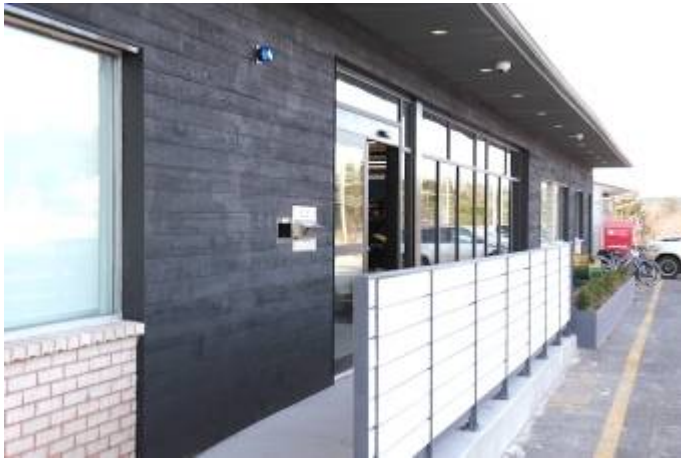
3.1 Halifax Public Libraries, Musquodoboit Branch.Exterior. Renovation, part of...
