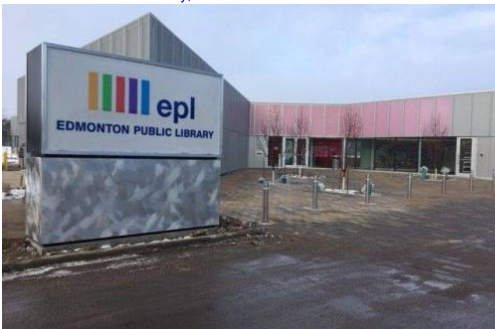
1.2 Edmonton Public Library, Calder Branch. Exterior. Credit Edmonton Public...
