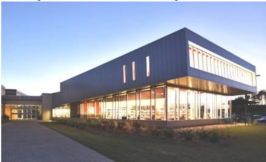
13.5 Vaughan Public Libraries, Pleasant Ridge Branch at night.Credit.Peter...
